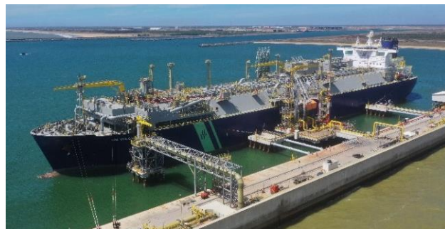
FSRU AT THE PORT OF AÇU. COURTESY BY GNA
