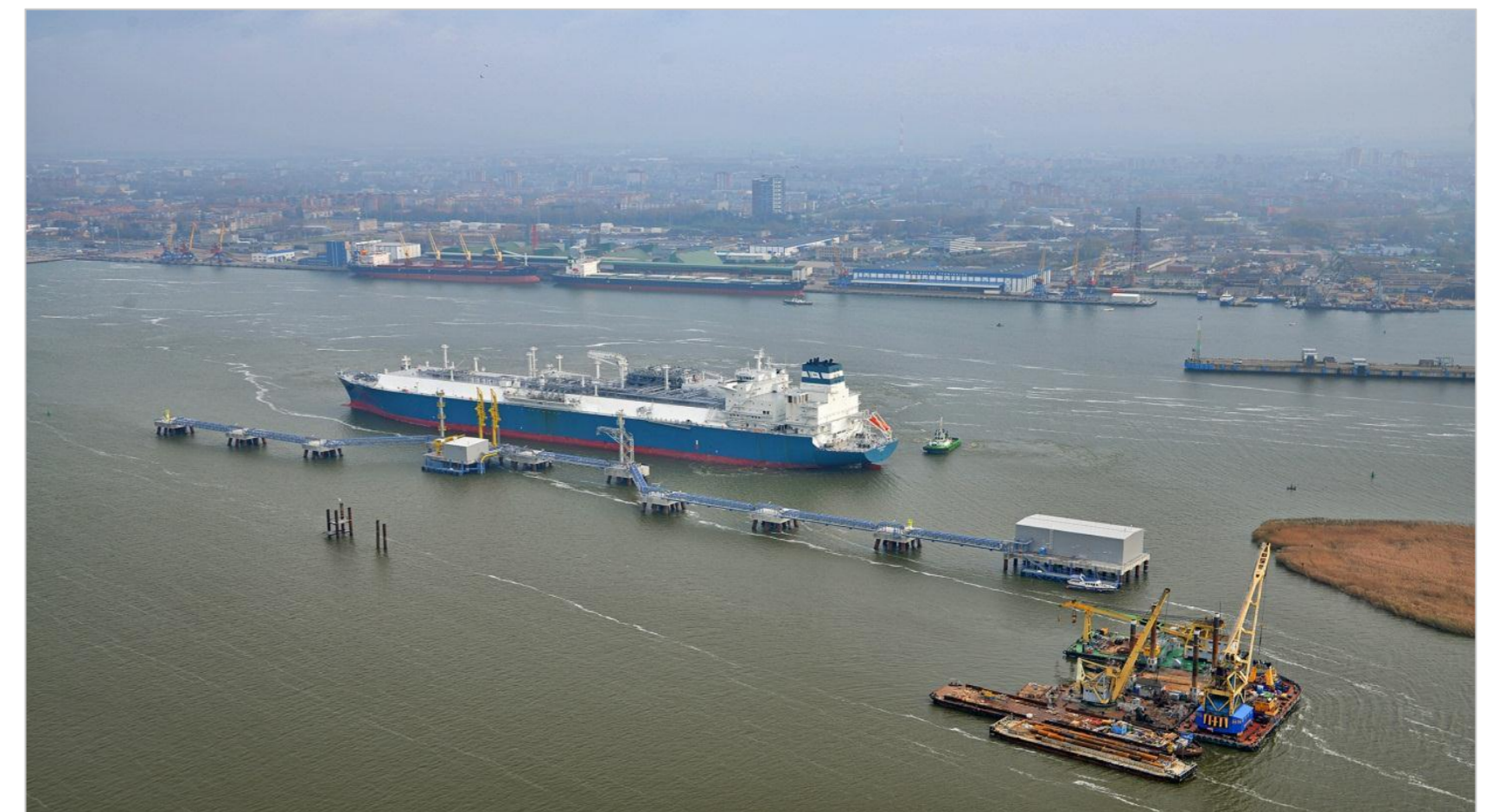
Liquefied natural gas (LNG) terminal
