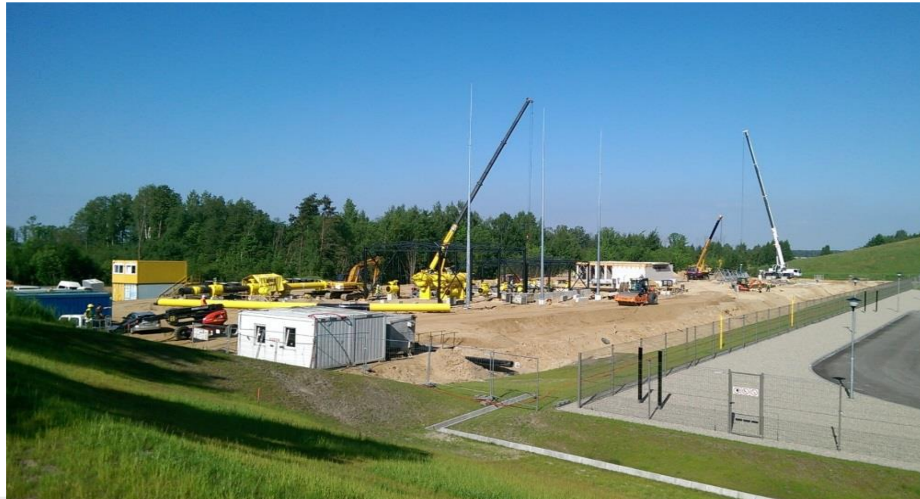
Gas metering station construction
