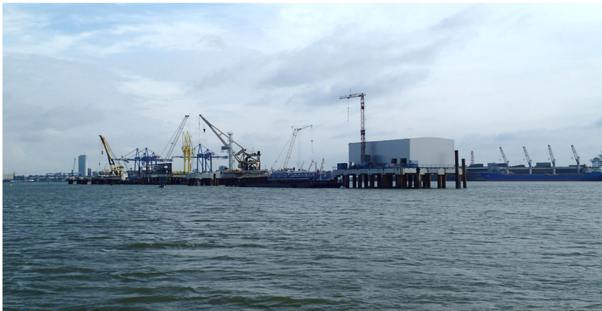
Jetty platforms concreting
