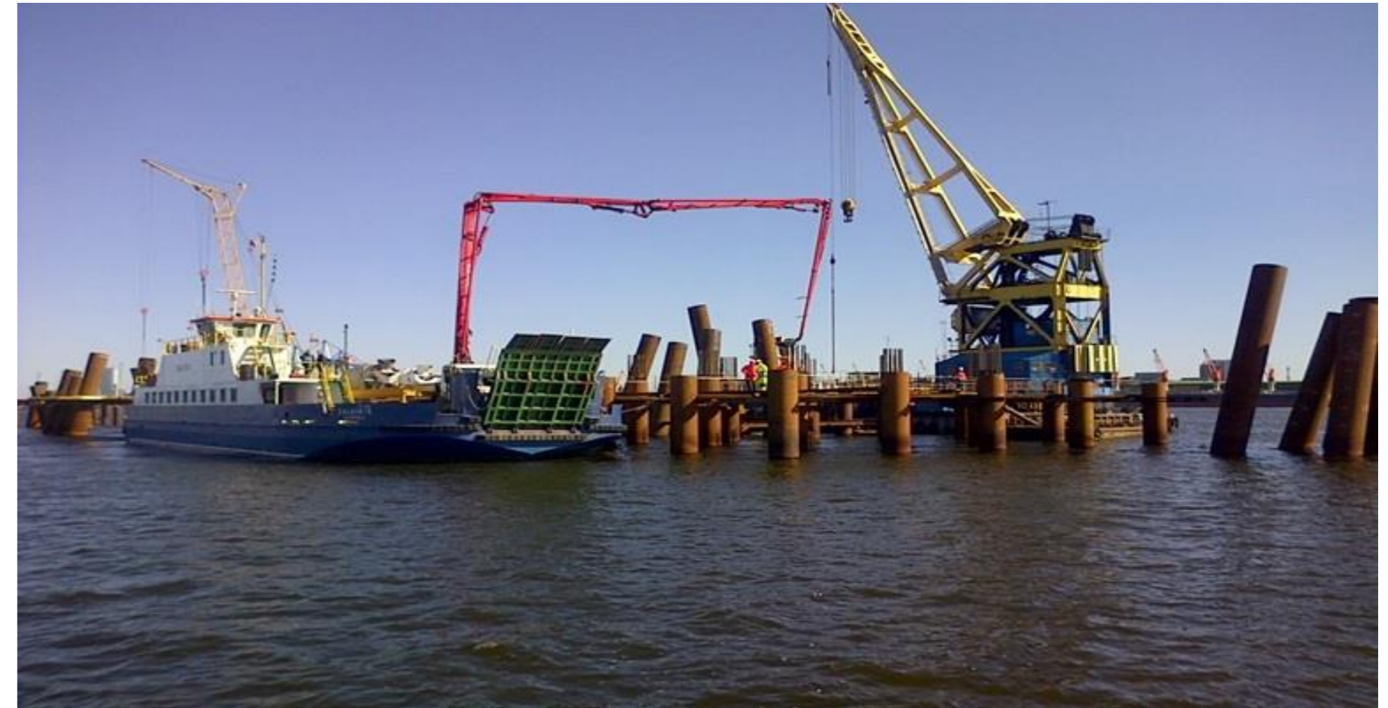
Piles concreting
