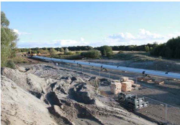
The Gas pipe line: views for the site
