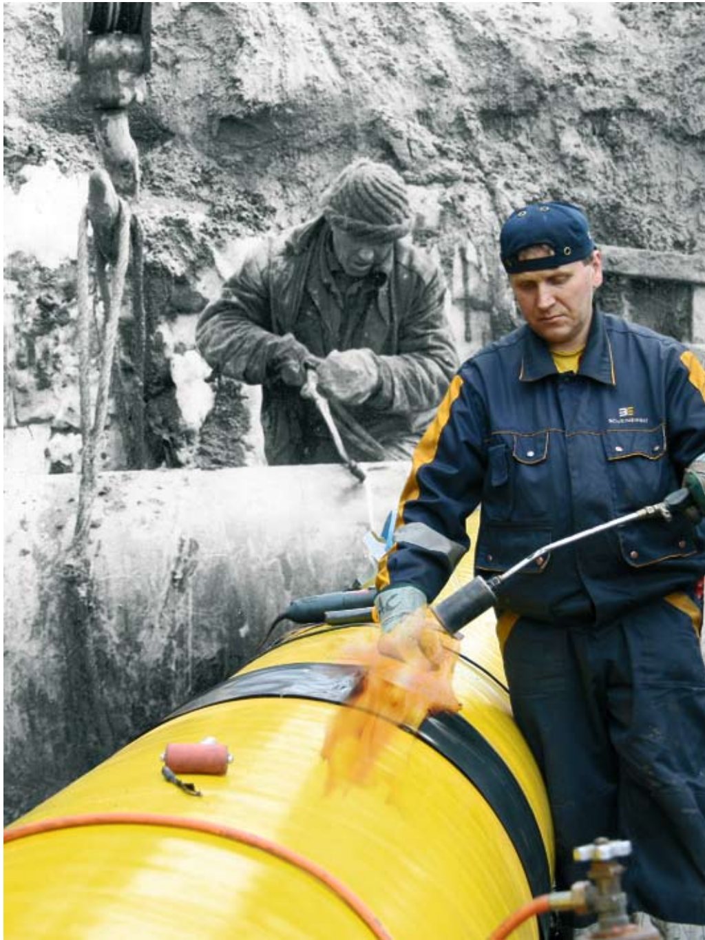
Construction of a gas pipeline, the years 1962 and 2007.
